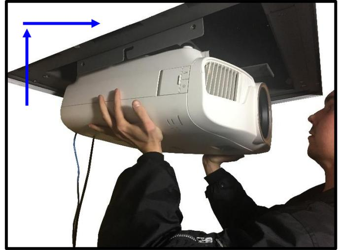
**Step 14:** Using the (4) Pre-Installed 3mm Hex Screws located on the Adjustment Bracket, fasten the Mounting Assembly to Crossmember. Again do not bump or move the Mounting Assembly until this step is complete.
