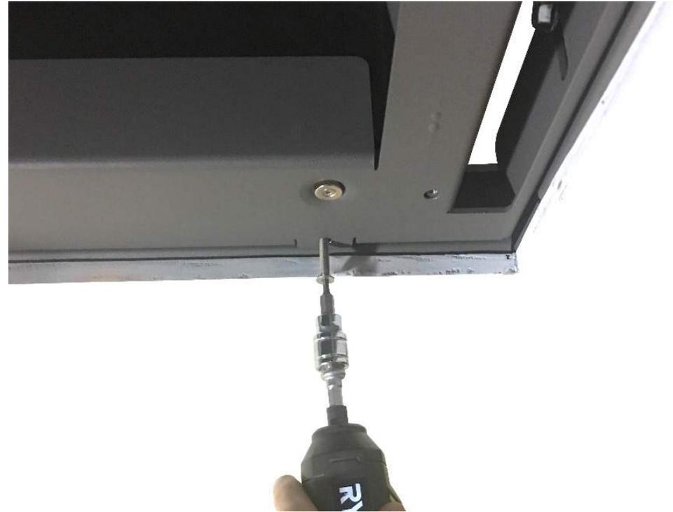
**Step 5:** Partially fasten the (4) Fine Adjustment Screws using the provided 1/8" T-Handle.
