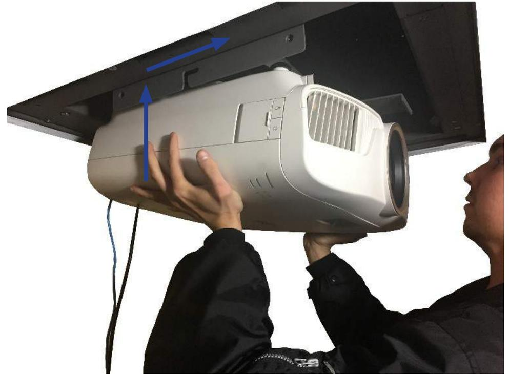
**Step 9:** Press the Shoulder Bolts on the Projector Mount into the keyed holes of the Crossmember, then slide it forward to lock it into place.
