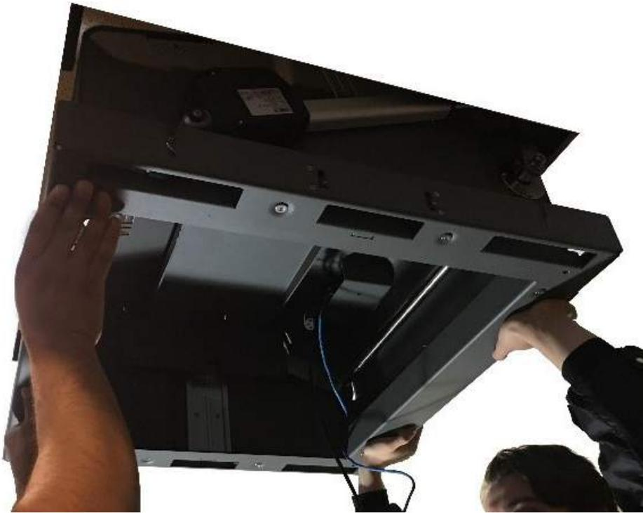
**Step 4:** Orient the E-550 Lift Mechanism so the front faces the direction you wish to project, then lift it up to snap it into the Installation Bracket.
