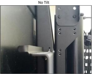
Step 29: Insert both Screen Locks into both Vertical Mounting Bars. Using (2) Screen Locks, place one Screen *Lock* on the bottom set of hooks for each *Vertical Mount* Bar. Using a Philips Head Screwdriver (not provided), tighten the Screen Locks against the bottom of the Screen Back Plate. This will ensure the TV does not slide left to right and eliminate the TV from being lifted off of the mount.
